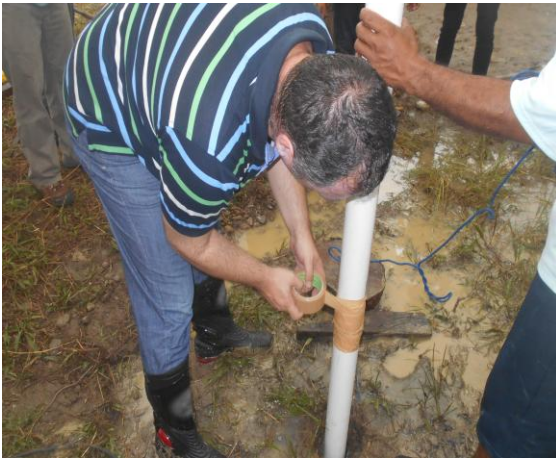
Fig.12:Pipes connection
