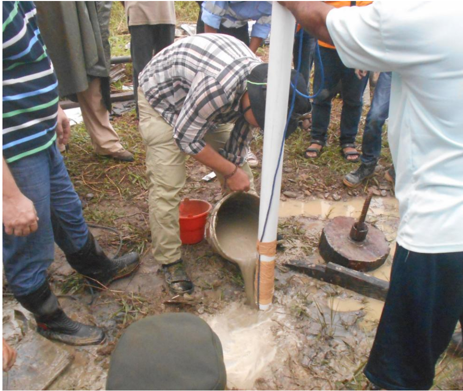
Fig.6: Cementation of the borehole
