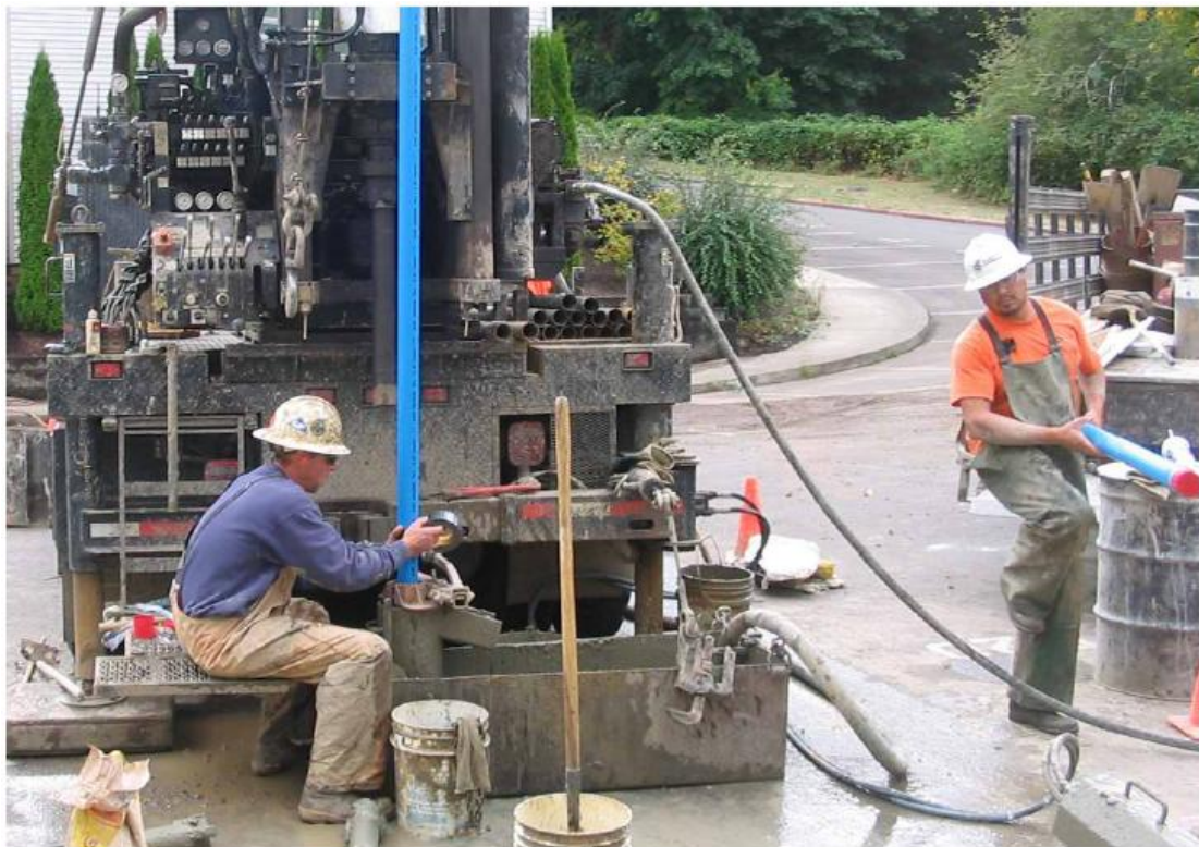
Figure 4: ABS casing installation
